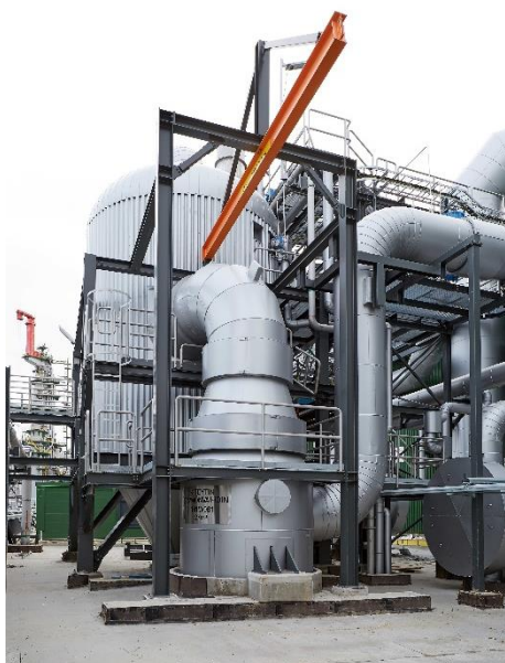
ANDRITZ has delivered several ARC systems for the removal of chlorides and potassium from the kraft chemical recovery cycle.
